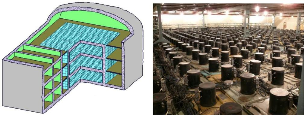
*Fig1. The Baksan Underground Scintillation Telescope, Right –the upper plane of the BUST*
